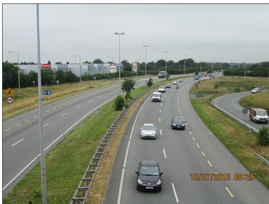
Plate 3.3: M7 at Maudlins Interchange
